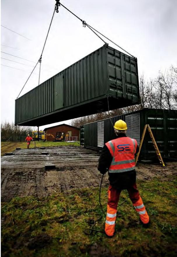
*Figure 18 SC and SLC each in a 40 feet container with step-up transformer, protection and control equipment is hoisted on to foundations at Hejnsvig 60/10 kV substation.*
