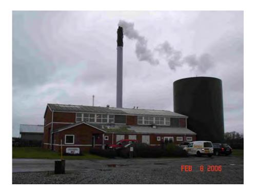
Figure 13 Hejnsvig CHP plant with hot water storage tank.
