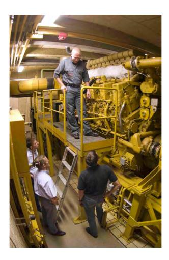
Figure 9 CHP plant natural gas engine.
