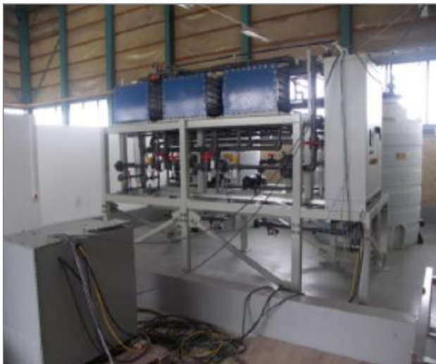
Figure 4.7: The Vanadium Redox battery in SYSLAB during installation and its system components (Source: DTU)
